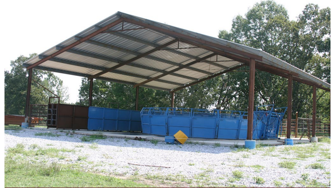
Figure 18. Covered cattle handling facilities.
