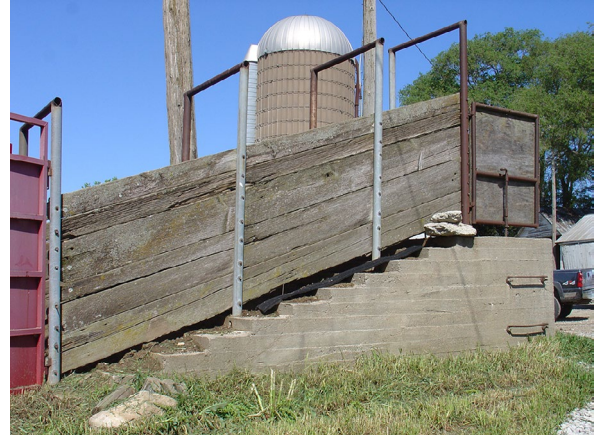
Figure 13. Permanently fixed loading ramps.
