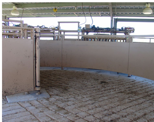
Figure 11. Textured concrete flooring in crowding pen area.
