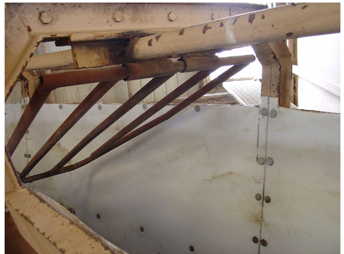
Figure 3. Backstop in alley.
