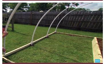
**Step 7:** Repeat the process to make and install the other three 20-foot bows on the remaining galvanized pipes.
