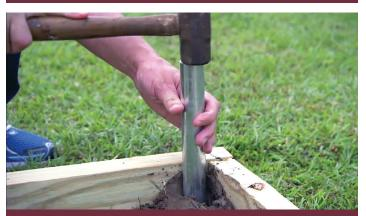
**Step 3:** Set the galvanized pipe using a hammer, leaving about 6 inches of pipe above the baseboards. At this point, you could use concrete to stabilize each post if you dug holes larger than the diameter of the galvanized pipe.
