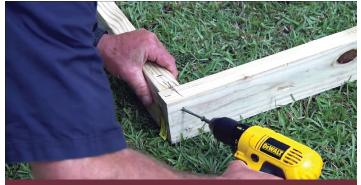
**Step 1:** Line up the 2x4-inch baseboards—two 10-foot boards and two 12-foot boards. Secure them with 2½-inch deck screws. (The 11 building instruction photos were provided by *Ask This Old House.*)
