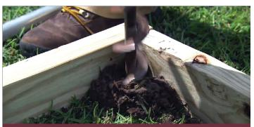
**Step 2:** Dig or drill holes for the eight pieces of galvanized pipe in each corner and along each long side to a depth of approximately 12 to 18 inches.
