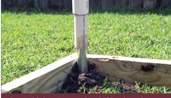
Step 5: Slide the PVC pipe onto the ends of the galvanized pipe.
