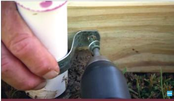
**Step 8:** Secure the PVC bows to the base using pipe straps and  $1\frac{1}{2}$ -inch deck screws.
