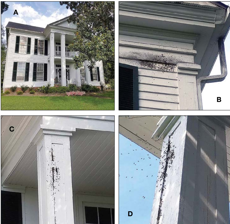
Figure 5. Here are several established honey bee colonies in cavities of a single house. A — Older homes tend to have more access ports for bees because of natural decay and settling of wooden structure that allows cracks and crevices to form. B — Staining of the wood identifies the entrance bees used to get behind the siding of the house to their colony in the hollow wall behind the façade. C and D — A colony of bees used this entrance to the tall, hollow columns of the porch. (Photos by J. W. Harris)
