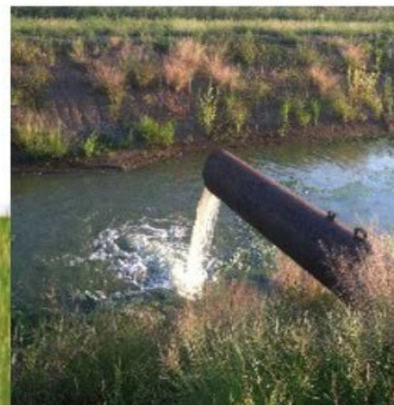
Figure 3. Above left: Receiving end of a riser board pipe. The boards slide along the grooves in the front of the pipe, which keeps water from entering the pipe. Above middle: Diagram of water flowing from a corn field on the left through a riser board pipe and into a TWR ditch. Notice the pipe is installed underneath a dike (pad). Above right: Water flowing from a riser board pipe into a TWR ditch.
