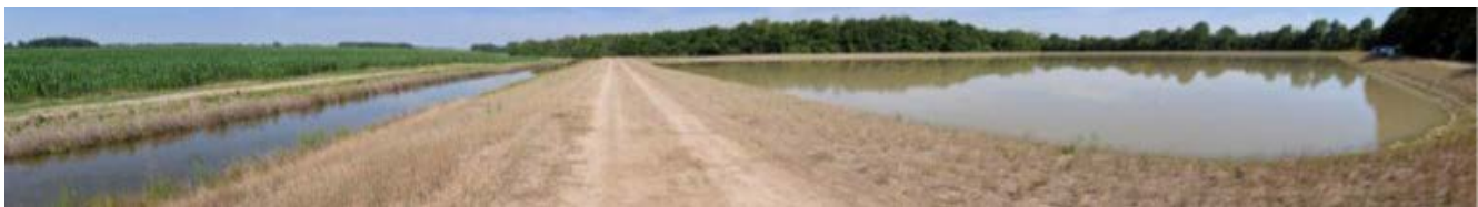
Figure 1. Top: Section view diagram of a TWR system installed in Mississippi’s Delta region. Middle: Plan view diagram of the same TWR system. Bottom: The TWR system shown in diagrams.
