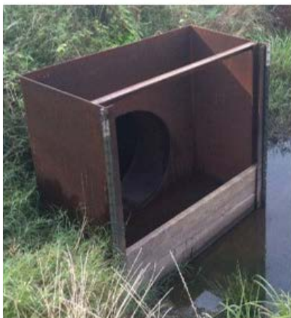
Figure 3. Above left: Receiving end of a riser board pipe. The boards slide along the grooves in the front of the pipe, which keeps water from entering the pipe. Above middle: Diagram of water flowing from a corn field on the left through a riser board pipe and into a TWR ditch. Notice the pipe is installed underneath a dike (pad). Above right: Water flowing from a riser board pipe into a TWR ditch.
